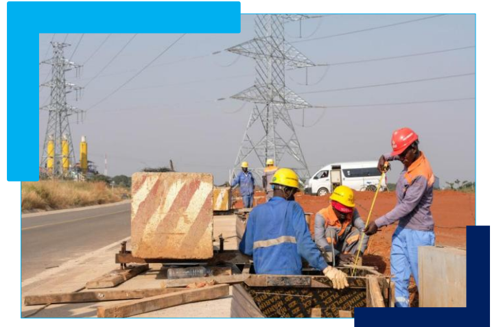
CONSTRUCTION OF CONCRETE TRAPEZOIDAL DRAINAGE
