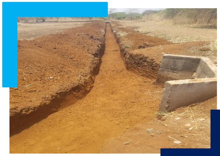
CONSTRUCTION OF SOIL TRAPEZOIDAL DRAINAGE
